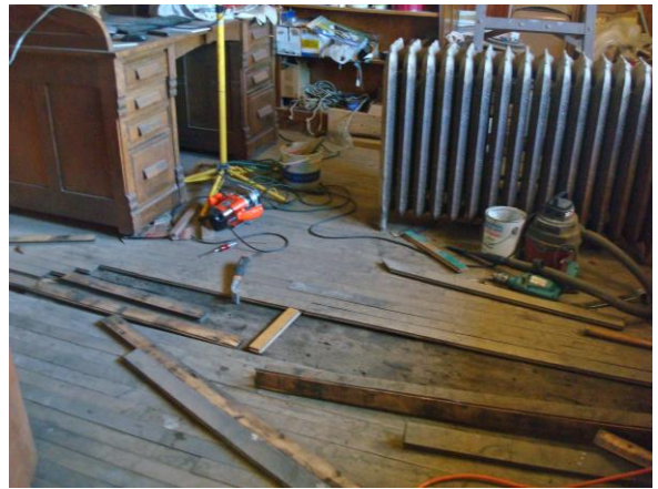
Smoking room at the depot as it was being worked on.
