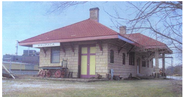
Waupaca depot. Restored Exterior and roof. Pftd.
